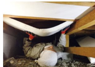
Achilles Juten R being installed
